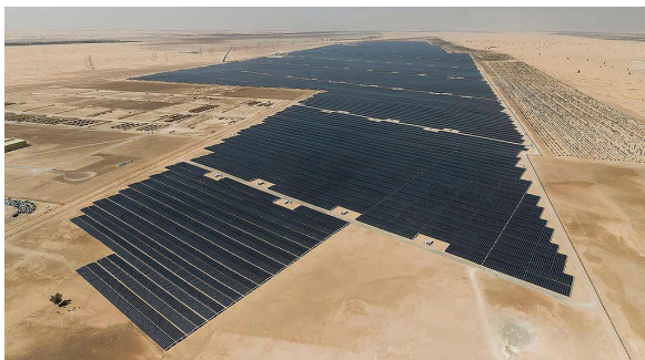
(a) Flat-terrain central-inverter plant.
